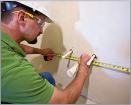
Field measuring for plumbing and electrical
