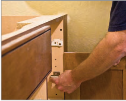
Doors adjusted on-site to ensure a proper fit
